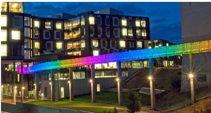
Figure 1. Lighting the Randy Pausch Bridge at CMU.
